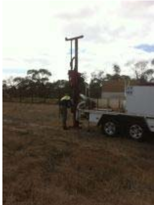
The soil-core drilling rig
